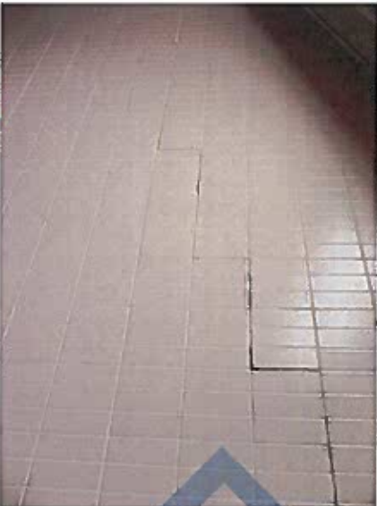
Figure 76- Stepped Crack in CMU Wall
