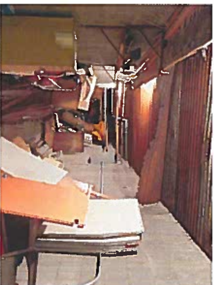
Figure 5- View of Underside of Ramped Walkway
