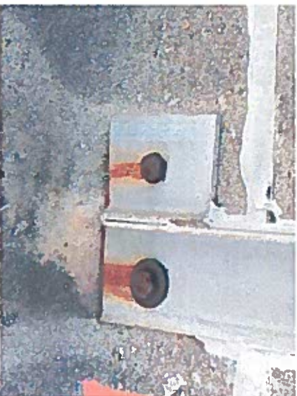
Figure 71 - Typical Seat to Precast Connection
