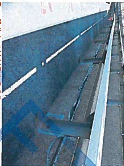
Figure 50- Horizontal Joint Sealant Failure
