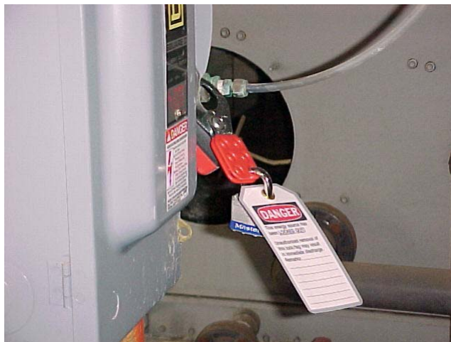
Typical Lockout/Tagout System
