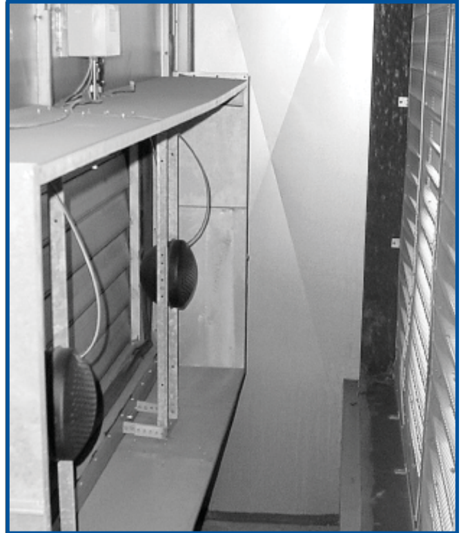
Probes Mounted Before a Damper
