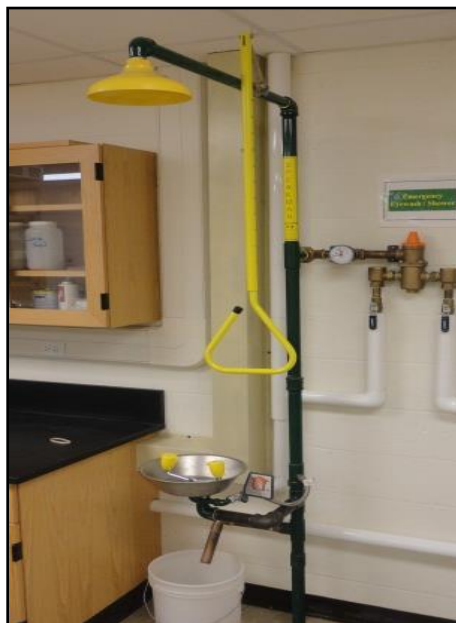
Examples of combination emergency eyewash/shower units
