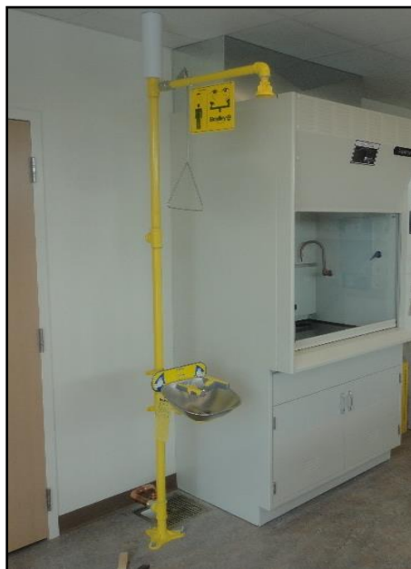
Examples of combination emergency eyewash/shower units
