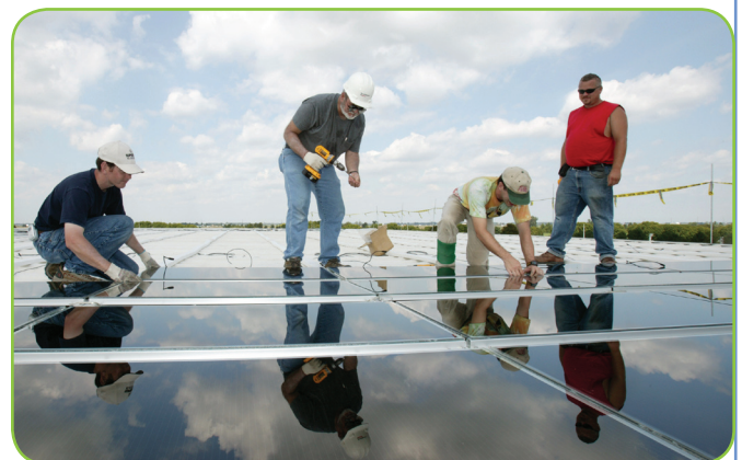
Photovoltaic panels being installed on the BGSU Ice Arena roof
