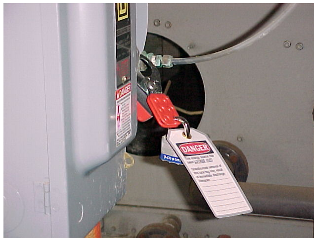
Typical Lockout/Tagout System
