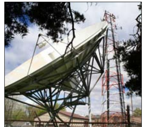
• One of the “dishes” behind the Tucker Telecommunications Center.
