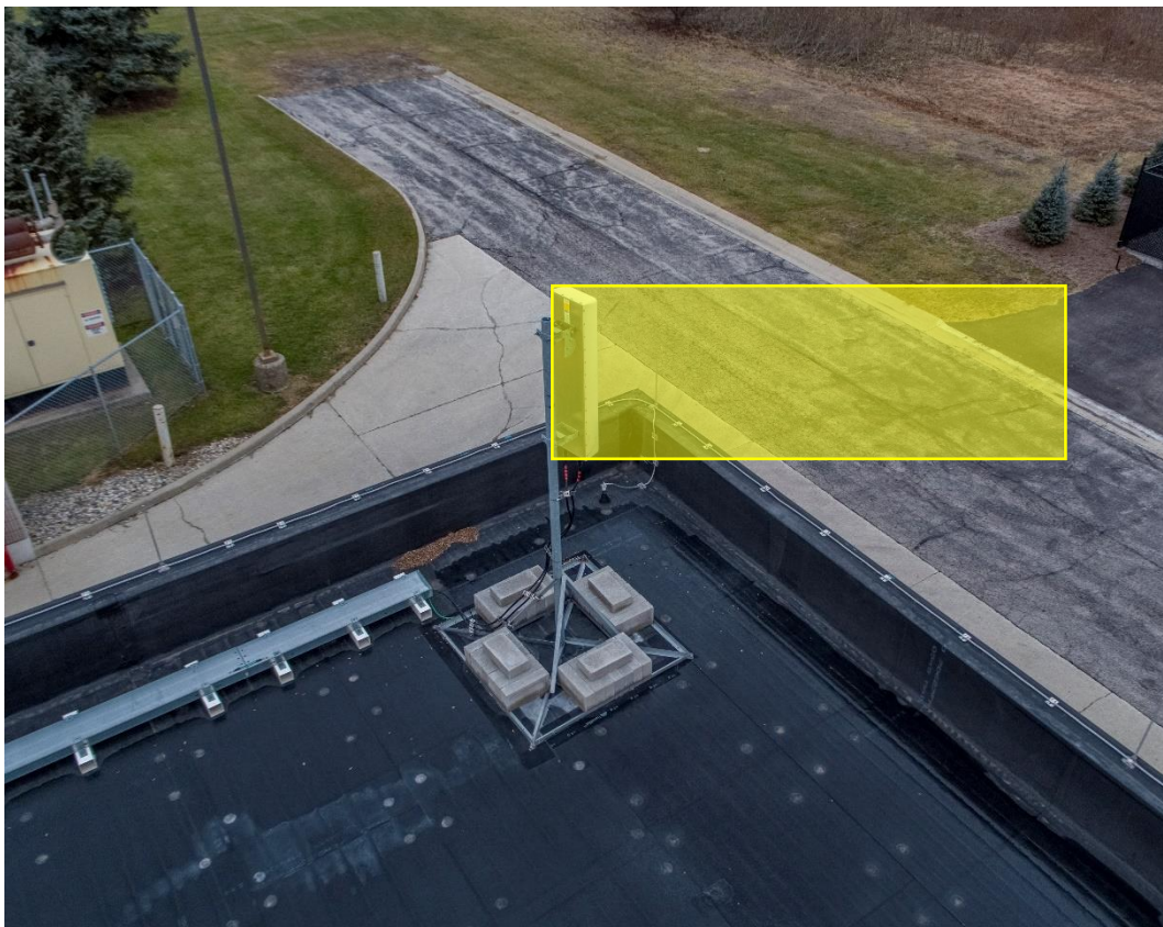
View of RF Device facing the North and the spatial RF hazard area.
