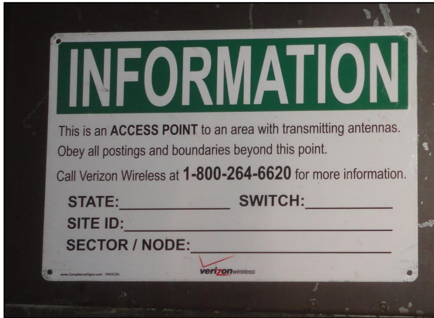
Figure 2: View of signage present that is meant to inform that there are transmitting antennas present beyond the sign. This sign may not be located near every piece of RF equipment as it is non-required.
