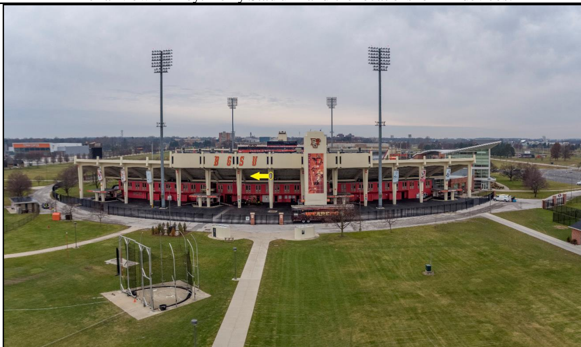
View of the East side of the stadium and the directional RF energy (from the East).
