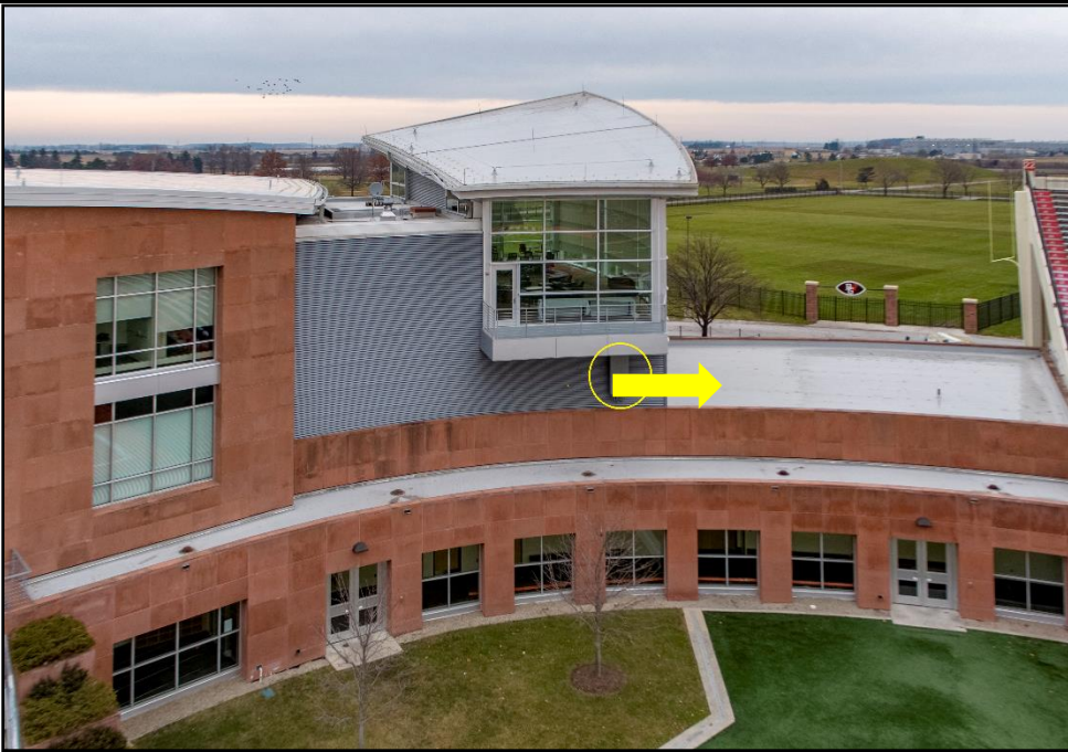
View of the Sebo Center RF device on the side of the building and the directional RF energy.
