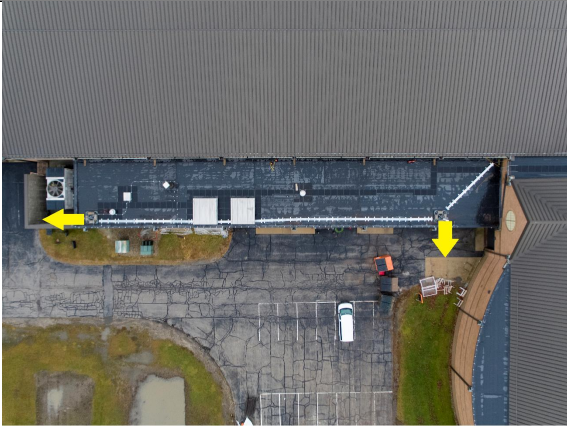
Aerial view of Perry Field House and locations of RF devices.
