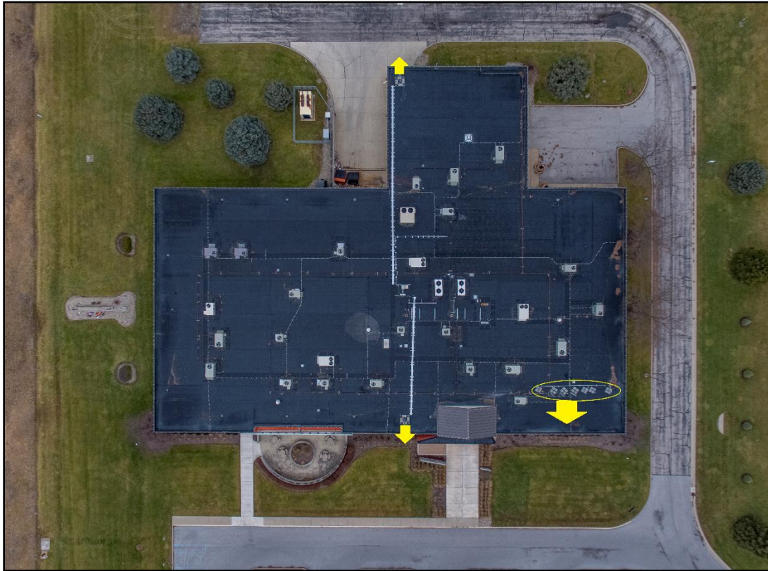
Aerial view of the Huntington Building and the directional RF energy.
