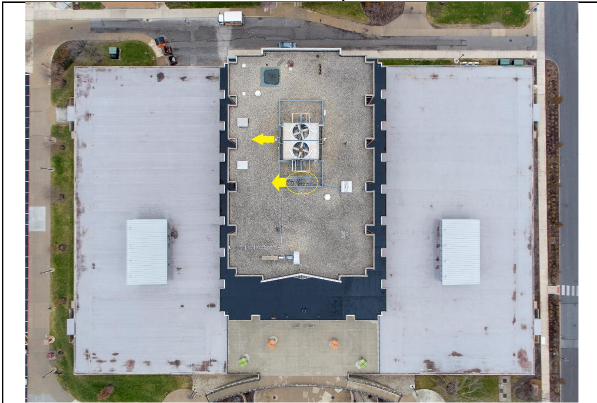
Aerial view of Jerome Library and the locations of RF devices.
