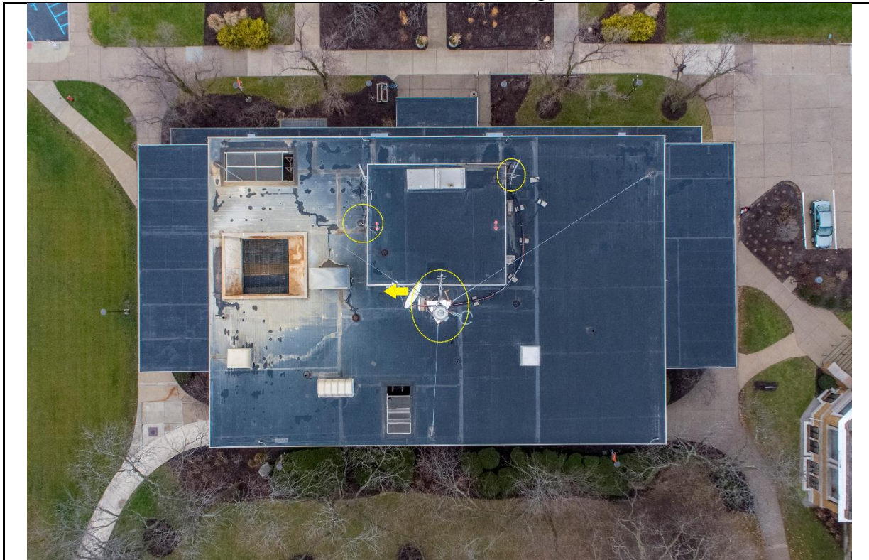
Aerial view of Administration Building rooftop with RF devices.
