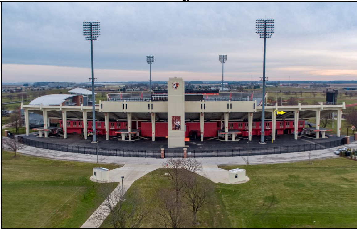
View from the West side of the stadium and the directional RF energy (from the West).
