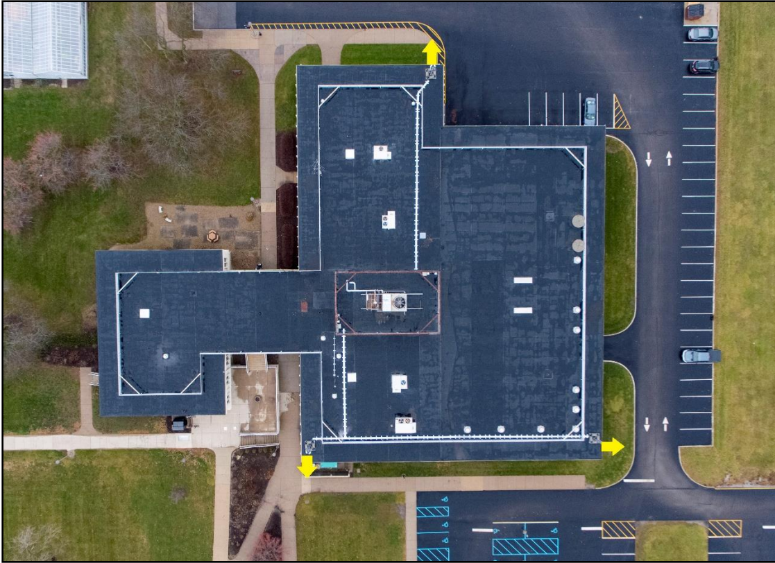
Arial view of Technology Building and the directional RF energy.
