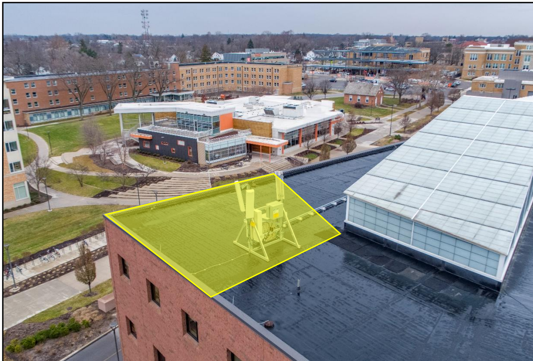
View of the RF source and spatial RF hazard area.
