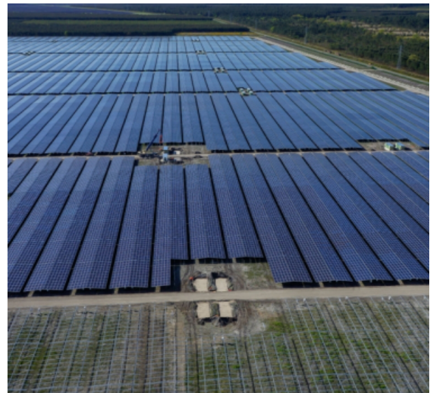
Figure 9. East/West Ground-Mount PV Array Configuration
