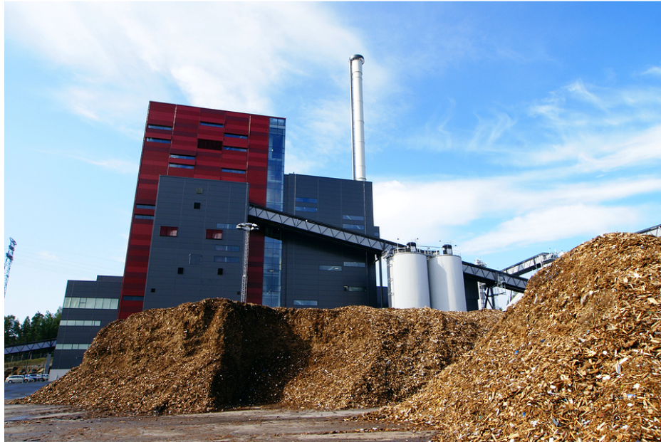
Biomass facilities can require lots of space for handling enormous amounts of woody waste.
