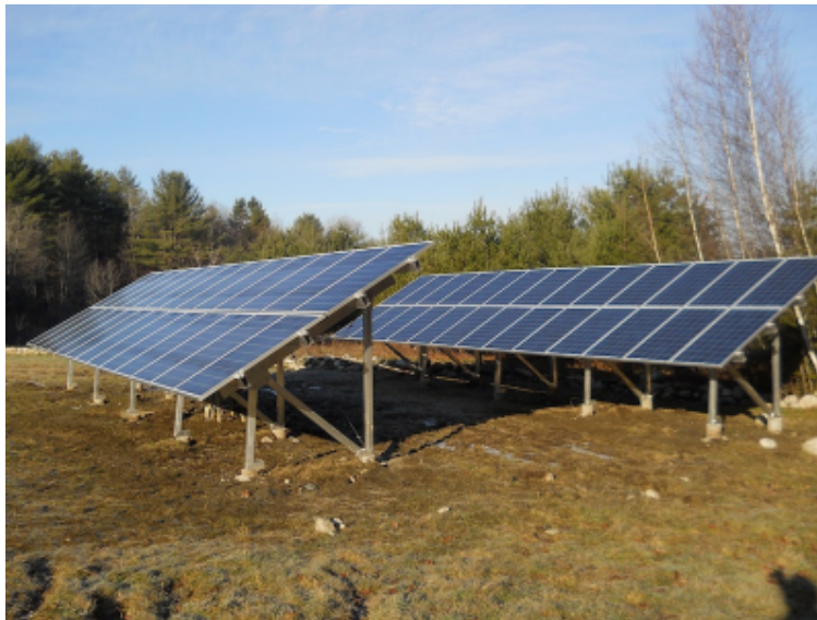
Figure 8. Typical Ground-Mount PV Array Configuration
